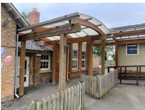
Fordingbridge Structures glulam timber / polycarb roof walker & shelter, 3 sections, 23x21ft / 42x11ft & 15x11ft
