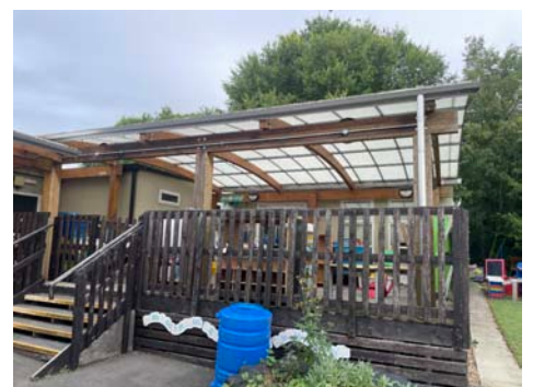
Fordingbridge Structures glulam timber / polycarb roof walker & shelter, 3 sections, 23x21ft / 42x11ft & 15x11ft
