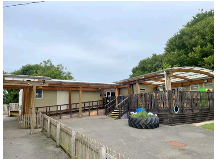
5x RLG Mobile Buildings (Elliot) 30x10ft modular cabins, 1x RLG Mobile Buildings (Elliot) 30x7ft 7" modular cabin, 3x RLG Mobile Buildings (Elliot) 28x10ft modular cabins & 2x RLG Mobile Buildings 19x10ft modular cabins configured:- 4x classrooms, library room, corridor / cloakroom, men / women / disabled toilets
