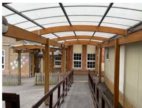
Fordingbridge Structures glulam timber / polycarb roof walker & shelter, 3 sections, 23x21ft / 42x11ft & 15x11ft
